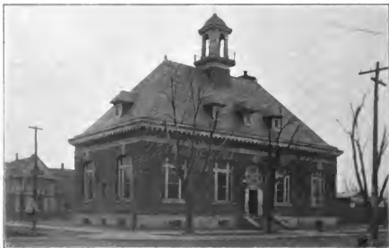
KIRKSVILLE POST OFFICE BUILDING.
